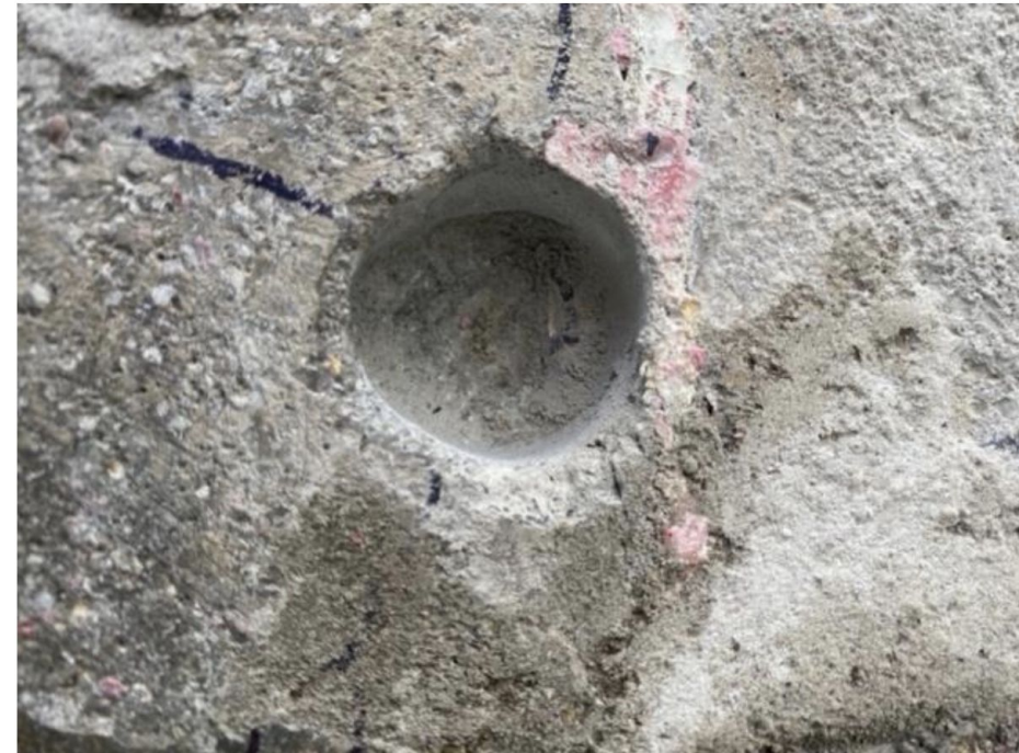
No evidence of corrosion risk at this location
