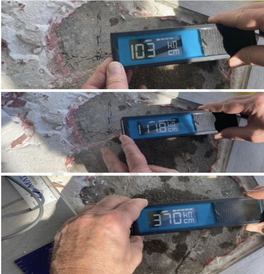
Concrete electrical resistivity measurement
